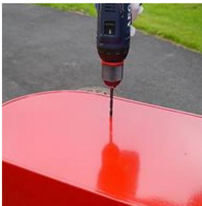
Place the letterbox face down onto the towel. Drill out the 4 preformed holes which are in the back of the letterbox.
