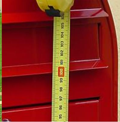
Ensure the height of the letter slot is approx. 1 meter from the ground.
