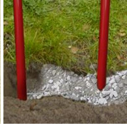
Fill the hole with coarse gravel or concrete.
